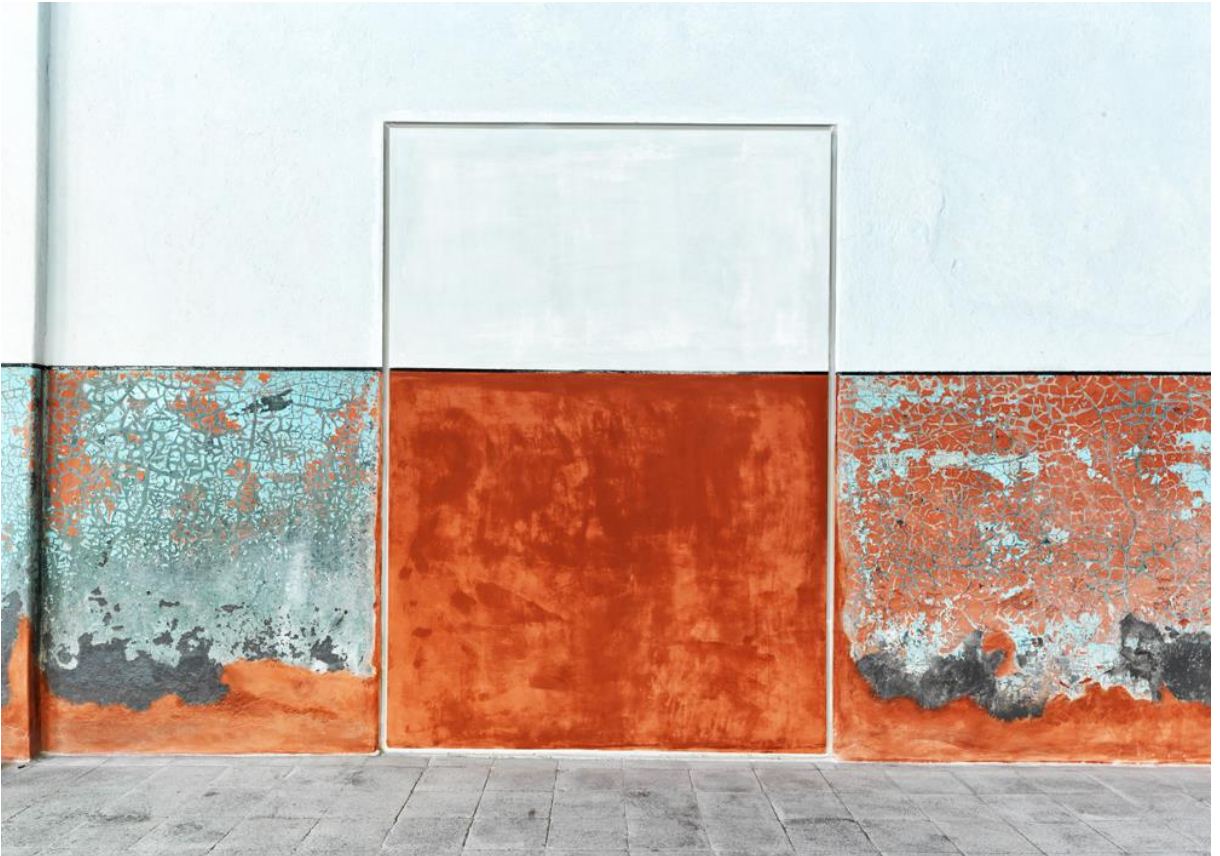
Image-4 Patina of walls after preservation
