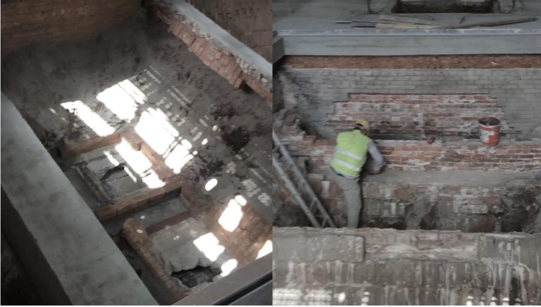
Image-1 Coal & Ash Chimneys before restoration
