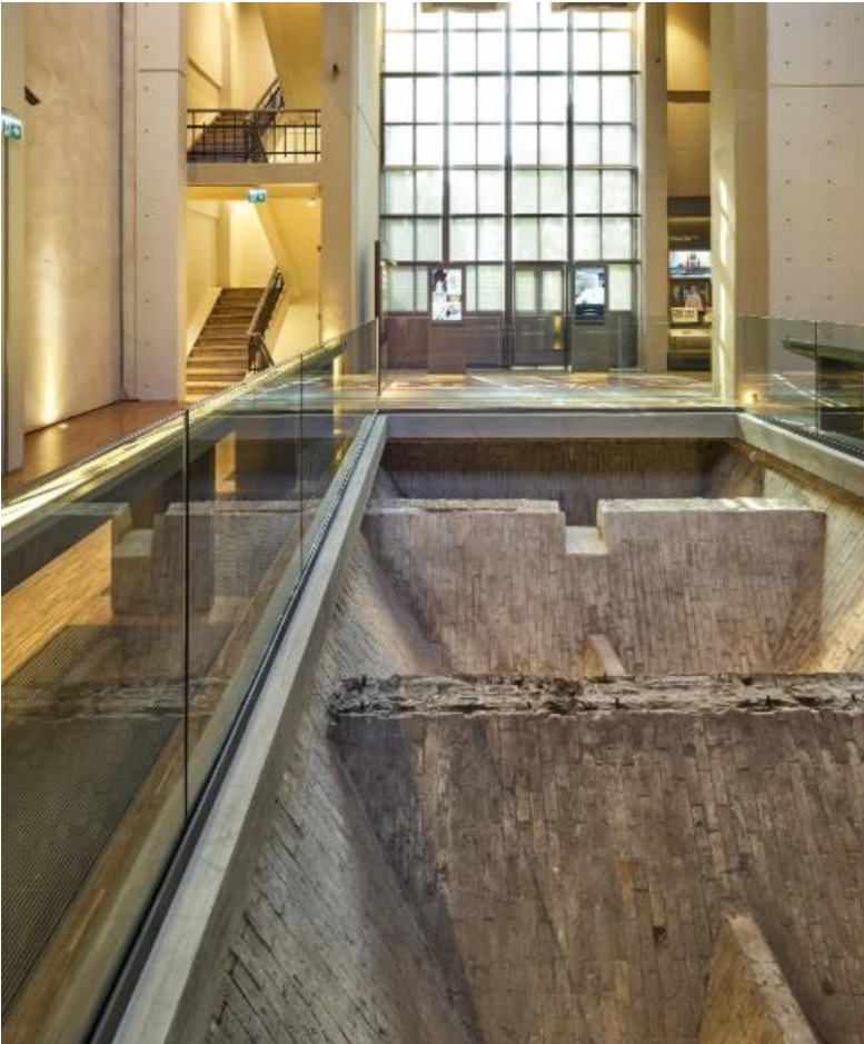
Image-2 Coal & Ash Chimneys after restoration
